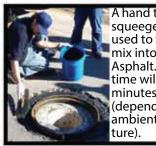
A hand trowel or squeegee maybe used to feather mix into existing Asphalt. Working time will be 5-8 minutes, (depending on ambient tempera
