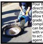
Pour the mix directly into affected area and allow to settle to grade. Empty pail completely. Tools can be sprayed with vegetable oil to act as a release
