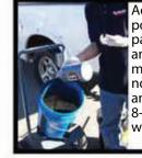
Add the B side polymer, place paddle in the pail and mix for 1 minute. The mix is now reactive with an approximate 8-10 minute working time.
